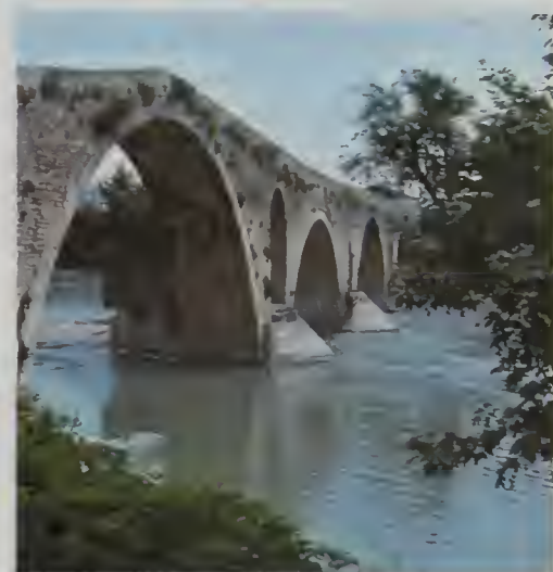
Seventeenth-century bridge over the Árakthos Potamós (river), Árta, Greece
